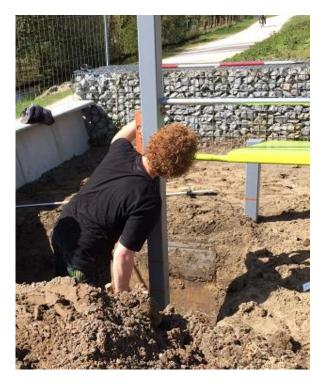
Tighten the security bolts completely **ONLY** when the posts are level and then close the hole with sand, at least until the dry sand level marking.
